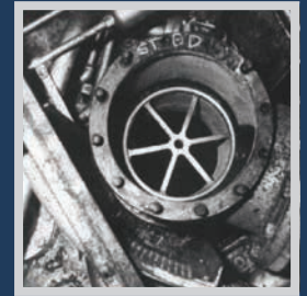
Main suction valve of sister ship after 9 months with MARELCO™ protection.
